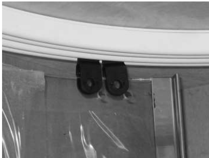
Fig 6: Position the door beneath the hangers.
