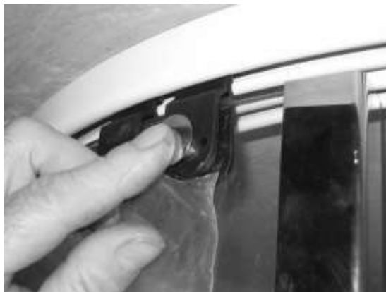
Fig 7: Fitting the interscrew
