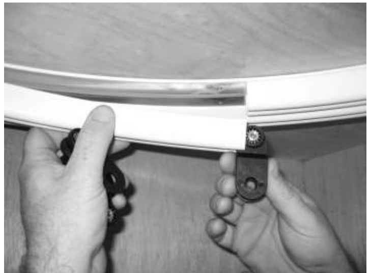
Fig 4: Lower the track to insert the hangers
